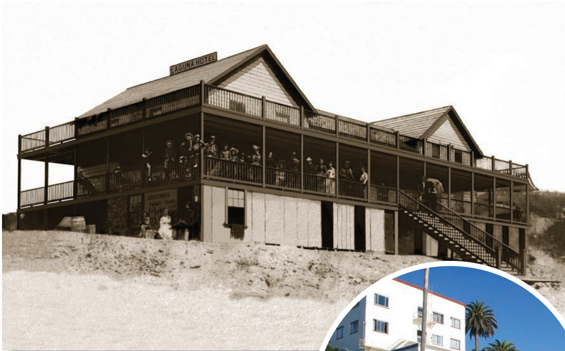
Above: Hotel Laguna was rebuilt two months after opening due to a fire (1888). Right: A present-day view
