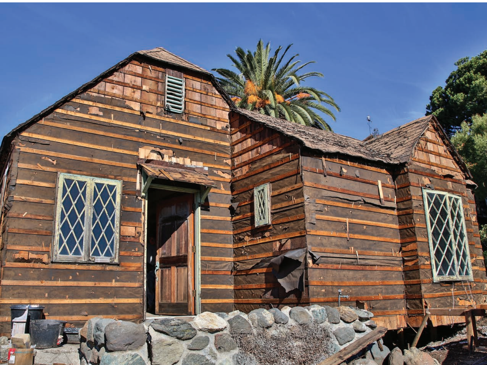
Local architect Bob A. McGraw and his team are currently working to restore this 1927 beach cottage on Wave Street.
